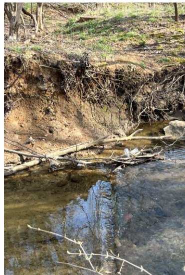
Eroded slopes along the banks.
