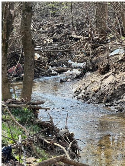
The channel has become blocked with debris (trees and trash)
