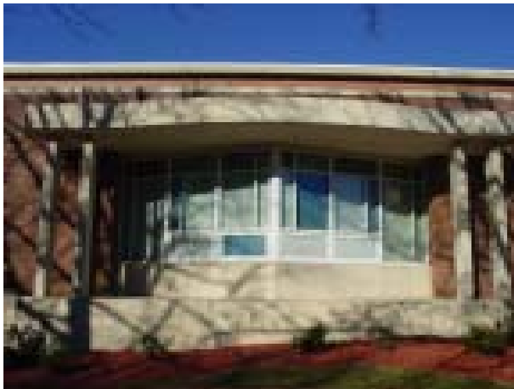
Window detail at Grandin Court Elementary School.
