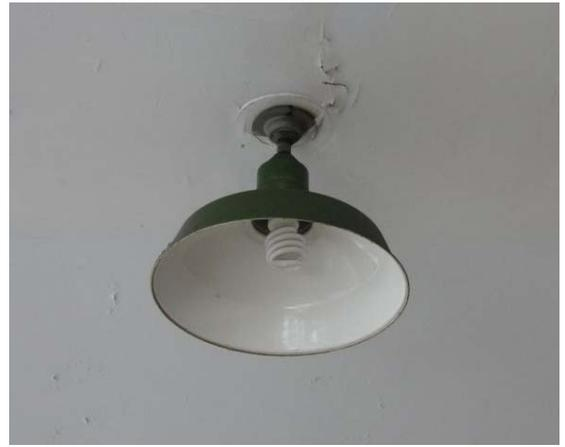
*The placement and design of this modern lighting fixture are inconspicuous and non-damaging to major building features. Additionally, the compact fluorescent light bulb in this fixture uses substantially less energy than a traditional incandescent bulb.*
