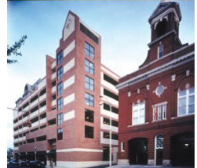
Century Station Parking Garage
