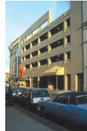
Center in the Square Parking Garage
