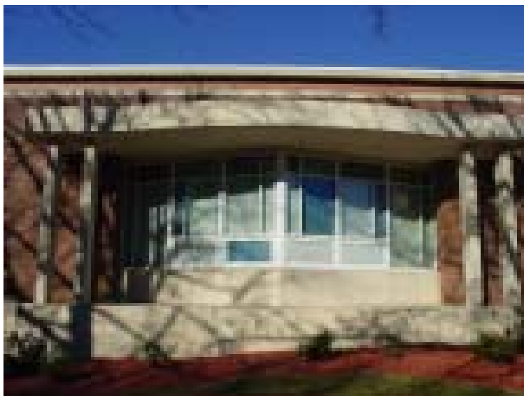
Window detail at Grandin Court Elementary School.
